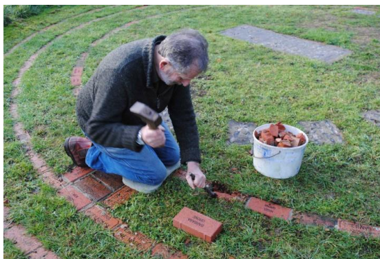
Pete lays one of the last new bricks, December 2018
