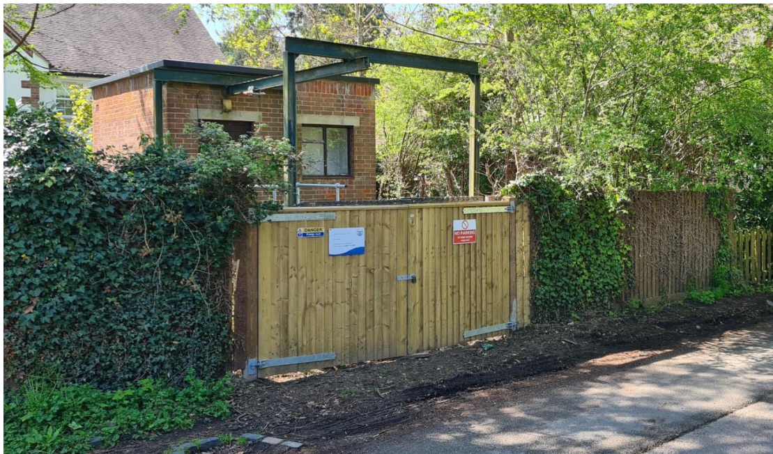
Eastfield Lane Sewage Pumping Station, ref EASTP5ZZ
