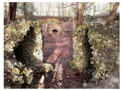
collapse of the chalk bank has now half-covered the tunnel entrance and made the icehouse inaccessible, as well as hazardous for visitors. However, the interior can still be seen from one angle *(below)*, revealing a domed circular chamber excavated within the
