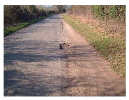
Unofficial passing place with road edge damage. Note the shallow entrance angle caused by vehicles gradually moving over without stopping, rather than turning into a lay-by. This is typical of the unofficial lay-bys. Similar erosion is occurring on the embanked section where for example the concrete fire hydrant marker which was on the road edge near Shepherds Close was lost in 2010.
