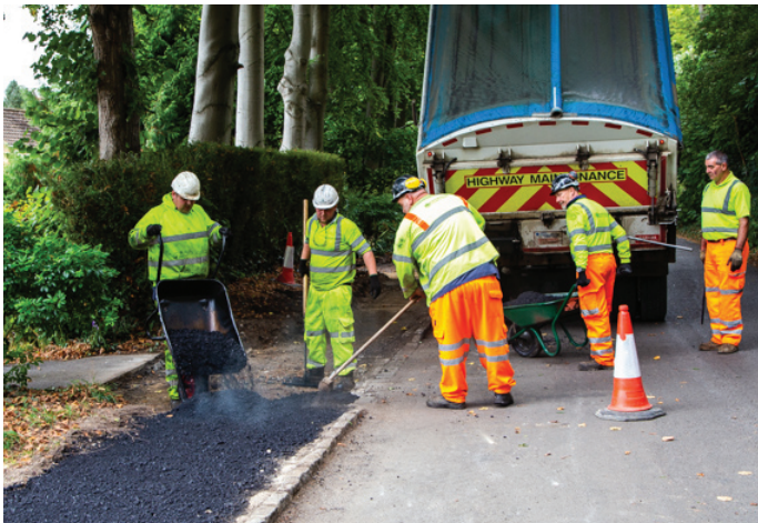
Contractors apply final layer to Hardwick Road pavement surface, photo courtesy Jim Donahue
