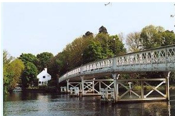
Construction began in late 1901 and finished in early 1902. The structure was gently arched and consisted of four spans with riveted lattice girders along the two outer edges; these acted as the main load bearing members and also as parapets. There were four 20 metre spans.
