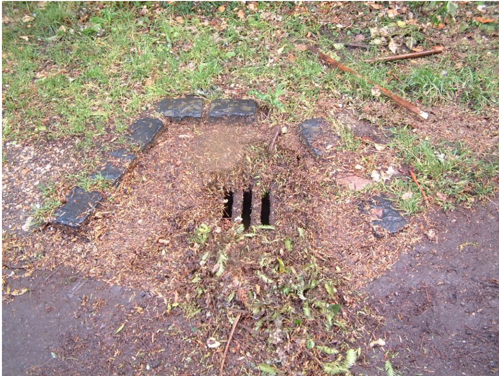
Figure 4 - A drainage gully after the storm. The leaf litter build-up, partly cleared by hand, can be seen. This gully is in Eastfield Lane.
