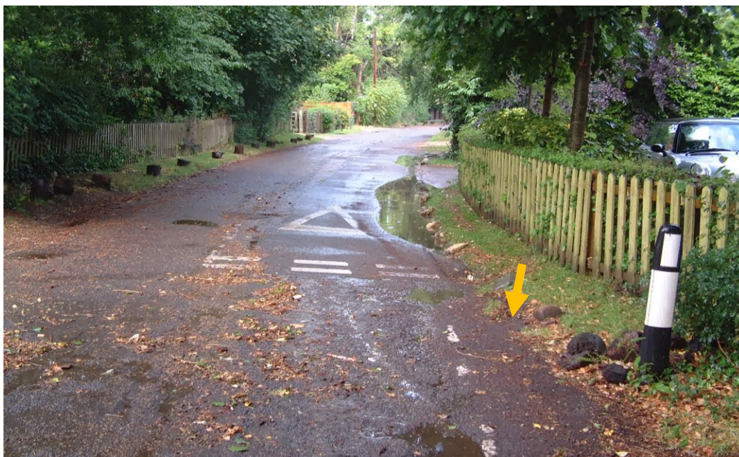
Figure 8 – After the storm, showing the road drainage gully (arrow) in Eastfield Lane, outside Chiltern Edge, which leads down to the culverted village watercourse.
