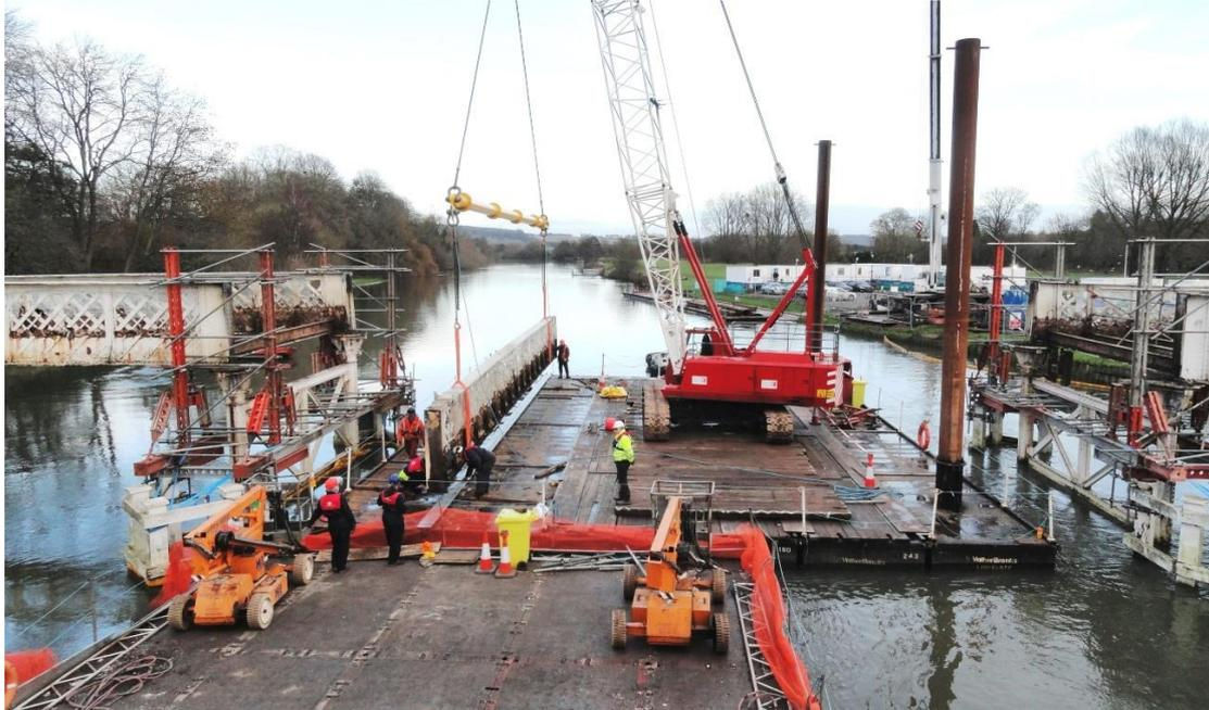
After a life of 111 years, the Whitchurch Toll Bridge crossing the River Thames was completely rebuilt in 2013-14. The new design was closely similar in appearance to the old, but with greater load-carrying capacity..
