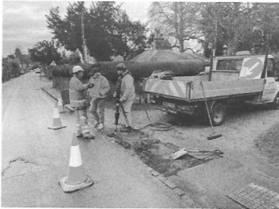
Work on High Street Wednesday.
