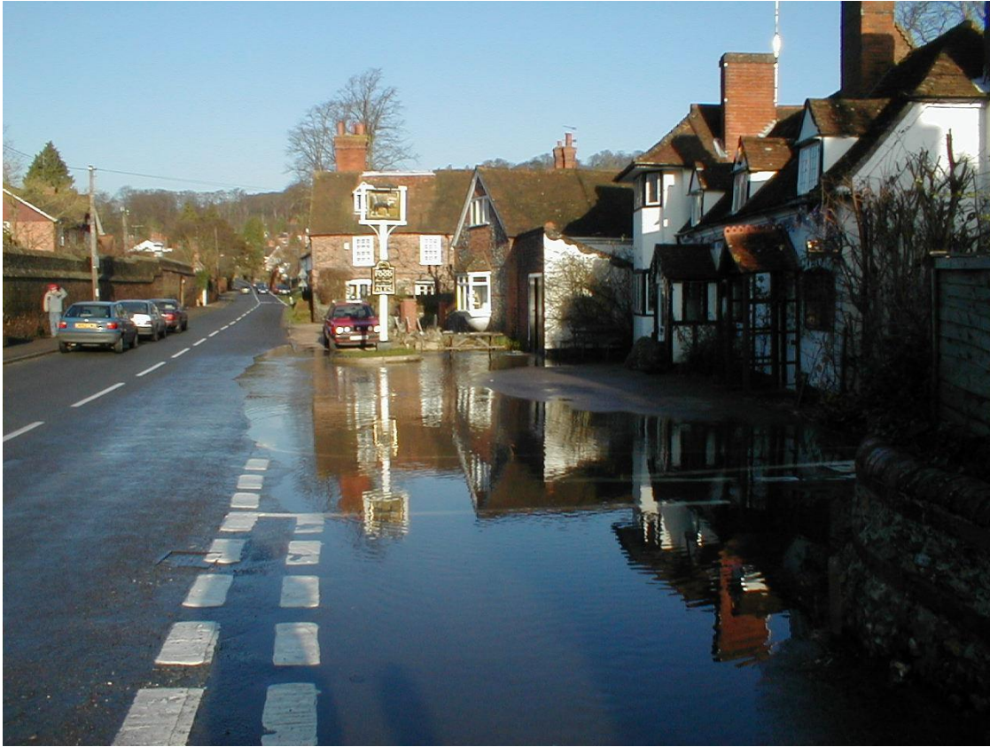
Figure 7 2003 flooding of The Greyhound - an undersized culvert south of Eastfield Lane could not cope with the flow of upstream height Thames water causing it to eject from a roadside drain in Eastfield Lane (to the right of the photo about 100 metres away)
