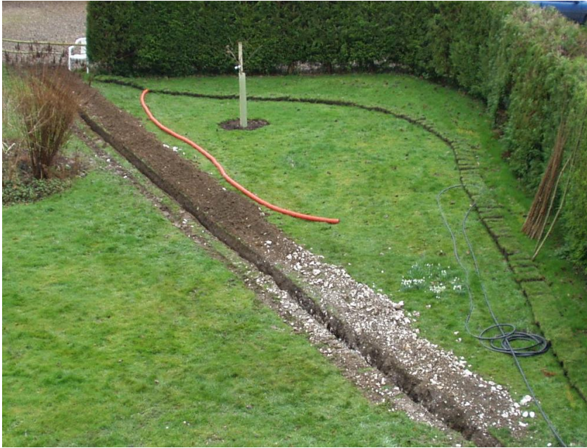
Figure 11 Chalk. This was used for the carriage drive and raised foundation of Thames Bank's new coach house.
