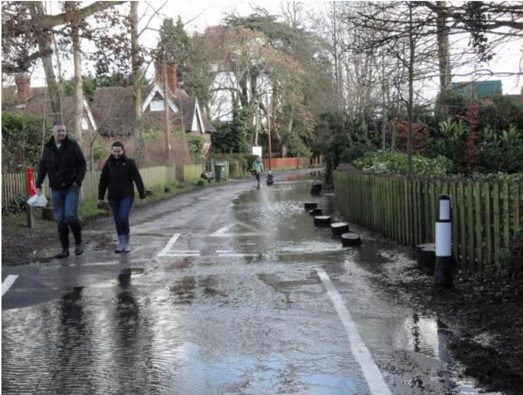
Figure 7. Flood water in Eastfield Lane, 10th January 2014. Note the tide mark to the north (left of photo) following the peak height at 9 pm the previous evening. This shows that virtually the entire road width was covered at the time of the peak.
