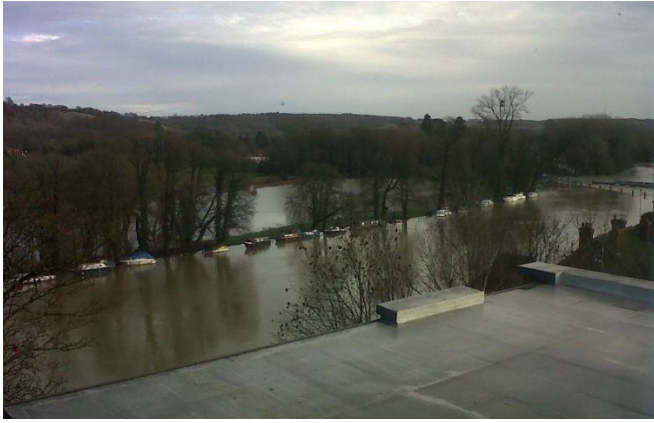
Figure 9 Walliscote farm's levee, overtopped 2014
