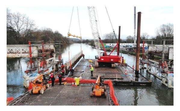
After a life of 111 years, the Whitchurch Toll Bridge crossing the River Thames was completely rebuilt in 2013-14. The new design was closely similar in appearance to the old, but with greater load-carrying capacity..
